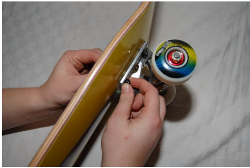
fig 33: Turn the nuts of the truck mounting bolts onto the truck mounting bolts by hand
